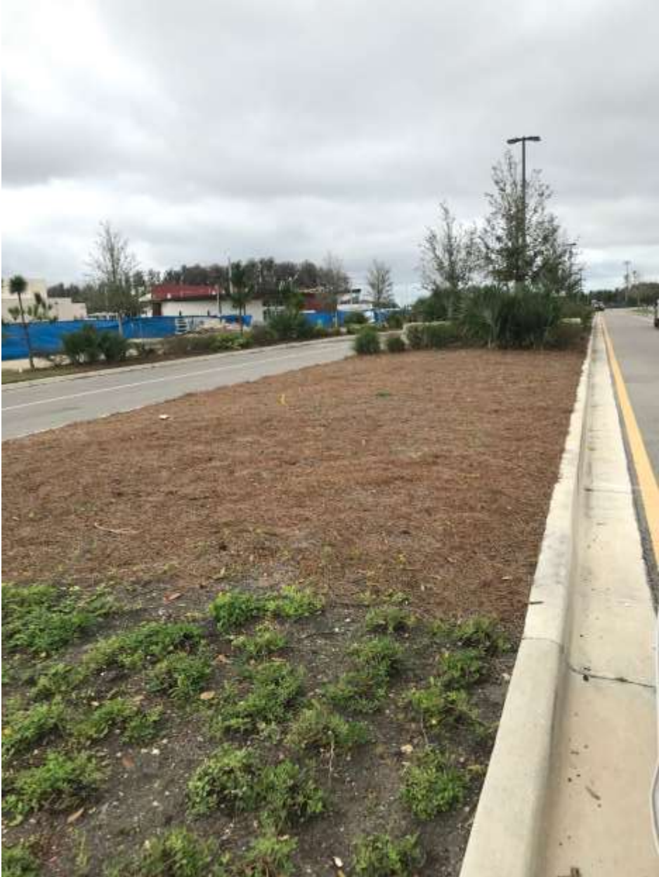
Estimate #4387 Lake Blanche, First median island at the Long Spur Lake Blanche intersection between the school and daycare construction. (Installation of Perennial Peanut to complete bed)
