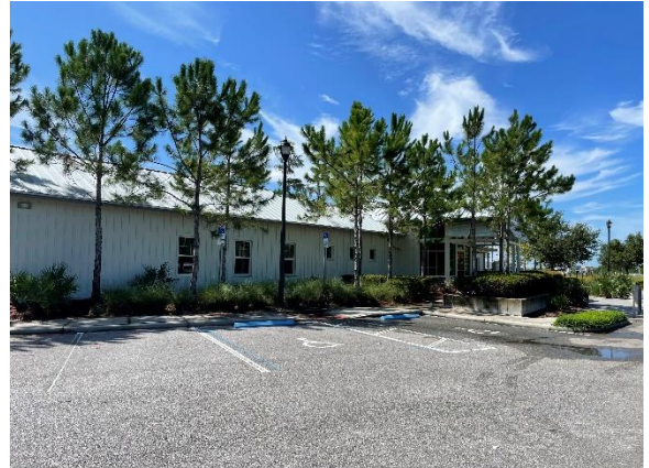
Exterior view of the subject property (Photo Taken on August 11, 2022)
