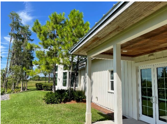
Exterior view of the subject property (Photo Taken on August 11, 2022)
