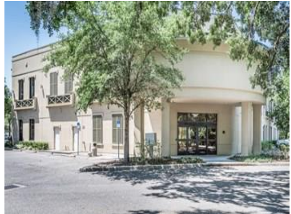
Lease 2 Barrister West
