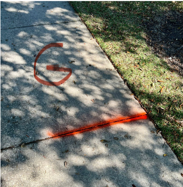
GRIND SIDEWALK SECTION AT CORNER OF RIDERS PASS/ LYON PINE LANE
