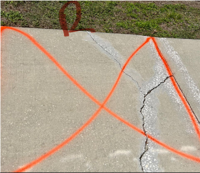
REPLACE SIDEWALK SECTION NEAR INTERSECTION OF HEART PINE AVE/ LONG SPUR
